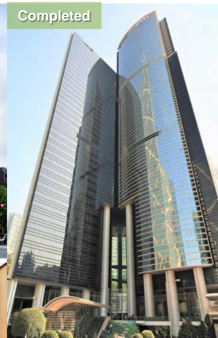
Three Garden Road ( Hong Kong ) 44 elevators
