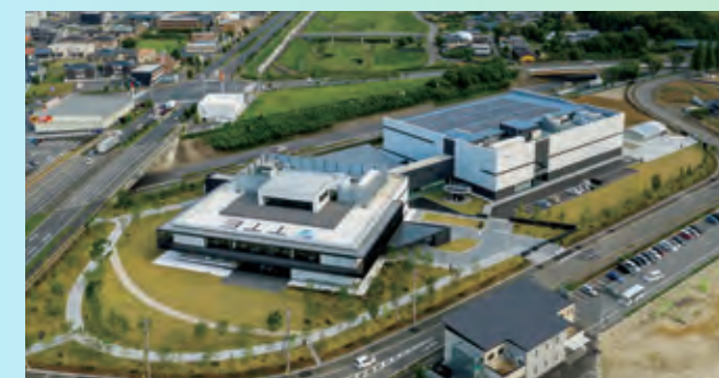
Takasago Thermal Engineering Innovation Center
