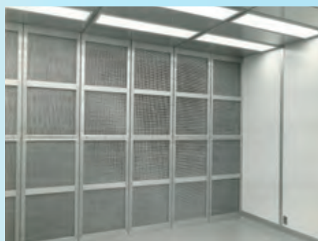
Takasago laminar flow cleanroom
