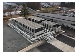
High-efficiency air-cooled modular chiller at the Okayama Plant
