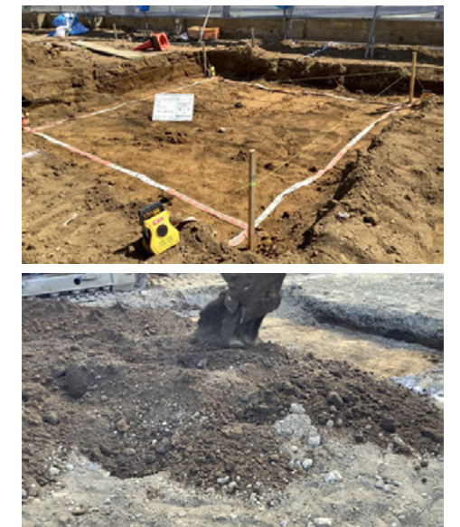
Top: Identification of the contaminated area Bottom: Replacement with healthy soil
