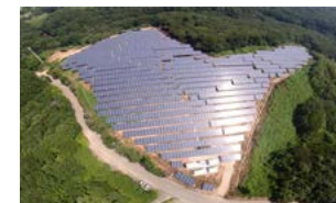
Hatoyama Solar Power Plant
