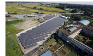
Oyama Solar Power Plant
