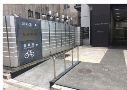
Creation of barrier-free access (Tenjin Prime)
