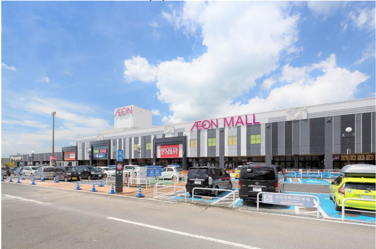
<AEON MALL Narita Photo of the Property >
