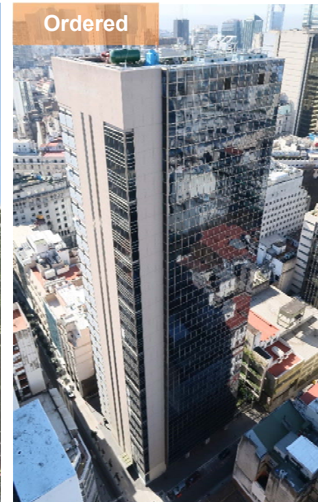
Maipu II (Buenos Aires, Argentina) Total of 9 elevators
