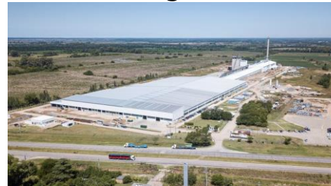
New float line in Argentina under construction
