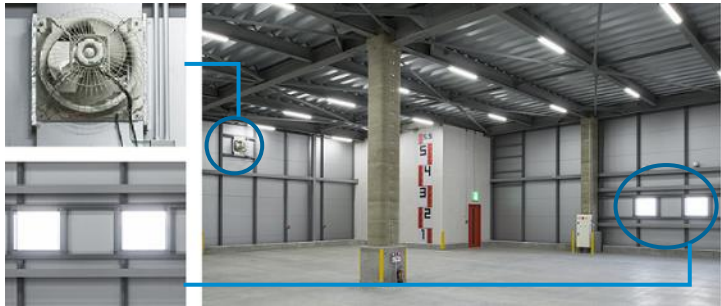
To help minimize costs in the future, the facility already has windows and ventilation built in to ensure compliance with laws and regulations in case it is necessary to expand office areas in the future.
