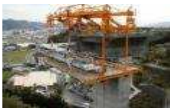
Shin-Tomei Expressway pier construction
