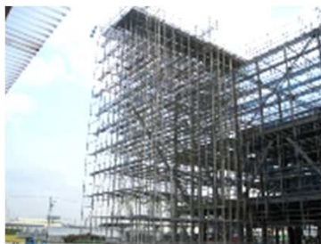
Large-scale warehouse/roof forming construction work
