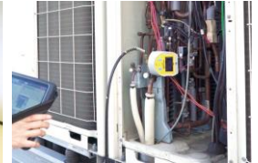
Pressure gauge connectivity
