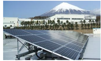
Fuji Plant (Fujinomiya)
