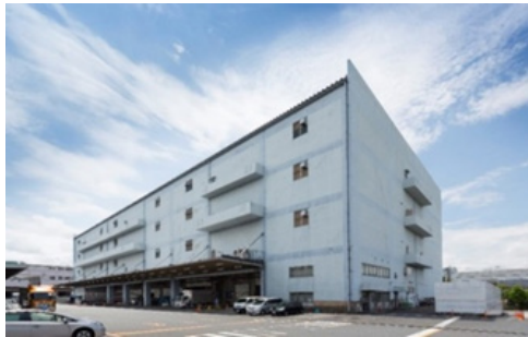
【IIF Yokkaichi Logistics Center ( Existing Building )】
