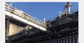
Muroran Works No. 5 coke oven (CO) refurbishment
