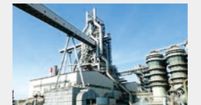
Kansai Works No. 2 blast furnace
