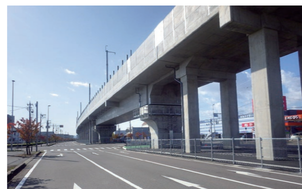
Hokuriku Shinkansen, Fukui Takayanagi Viaduct, etc.
