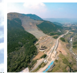
2017 Aso Ohashi Bridge Area slope disaster prevention construction
