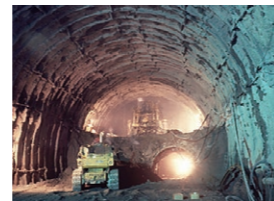
1977 Opening of the Joetsu Shinkansen Nakayama Tunnel
