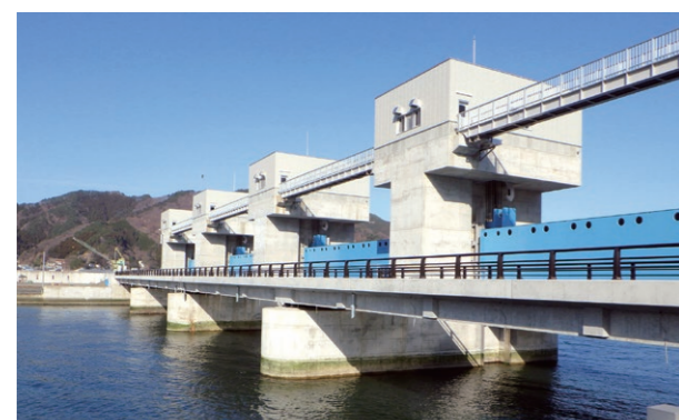
Class B river Kasshi River course Kasshi River floodgate civil engineering project
