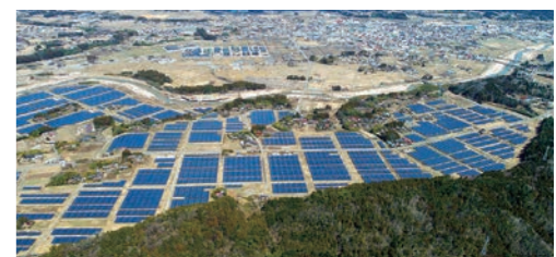
Namie Sakai Solar Power Plant 1 and 2 (Fukushima, Namie) (2020)
