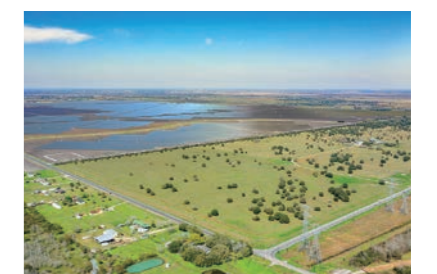
Solar Power Plants in Texas
