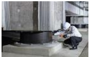
Seismic isolation structure
