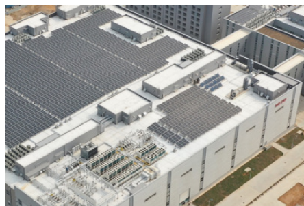
Photo 2: Solar panels installed on the roof
