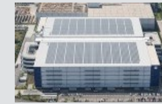
Solar panels for renewable energy utilization
