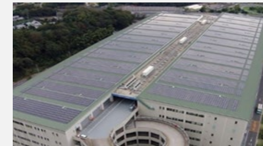
Installation of solar panels
