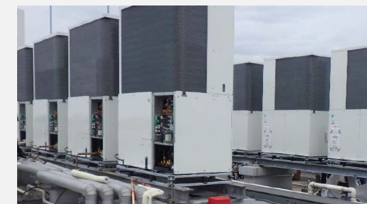
Installation of new air conditioning equipment
