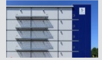
Exterior walls, sandwich panel system for thermal insulation and airtightness.
