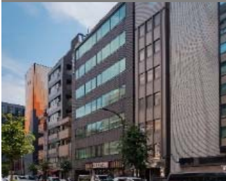
XYMAX Nishi-Shimbashi Building
