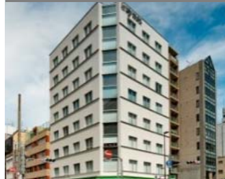
XYMAX Higashi-Ueno Building
