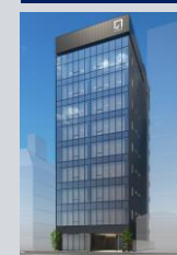
S-GATE FIT Hatchobori
