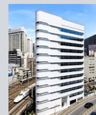
X-PRESS YURAKUCHO BLDG. managed by S-GATE
