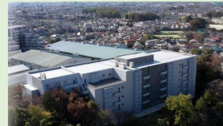
The 1st Tokyo Distribution Center
