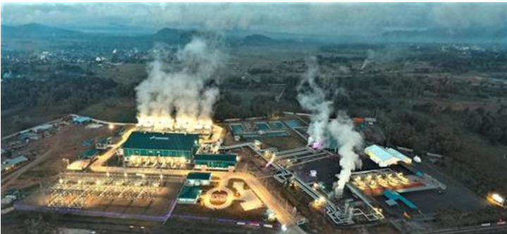
Control system and integration service order for Lahendong geothermal power plant in Indonesia
