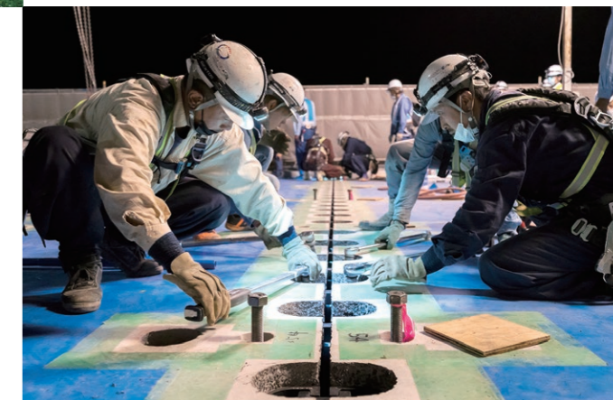
Connecting the joints
