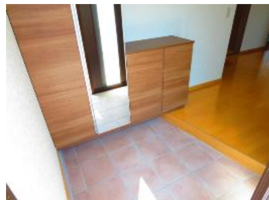
Renovated entrance, by replacing the carpet with flooring, cladding the entrance foyer with new terracotta-style tiles and installing a new shoe closet
