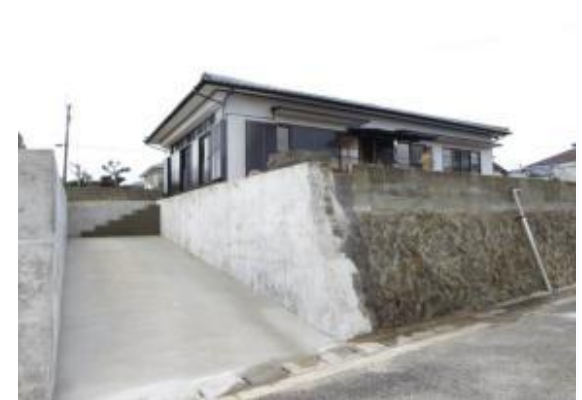
House where two parking spaces were created by removing garden trees and part of the retaining wall
