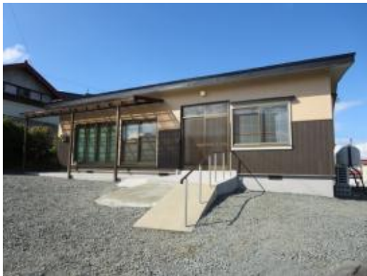
Renovated one-story house: replaced the damaged eaves and refreshed the dilapidated exterior
