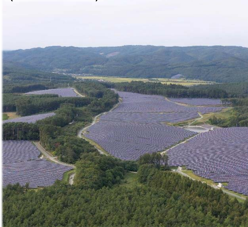
View of site (As of October 2021)
