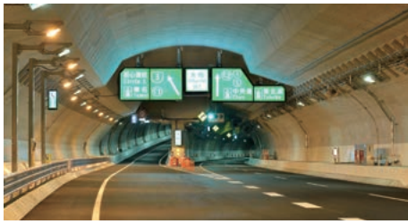
Ohashi Junction to the Shinagawa Route on the Shuto Expressway Central Circular Route (C2) (Tokyo) 2014
