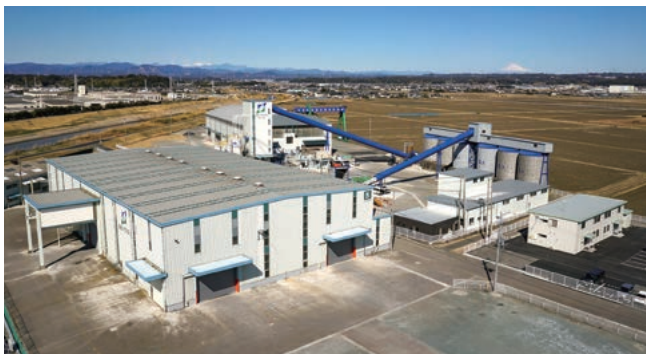
The new Kikugawa Plant.
