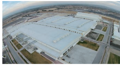
Honda de Mexico Transmission Plant (Mexico) 2014
