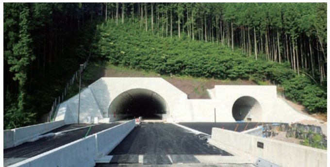
Completed shaft entrance.
