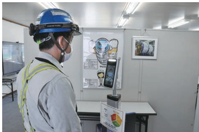
A new construction management service to manage work site entry and exit is being tested (it also checks body temperature).
