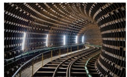
Curved section of the shield tunnel.
