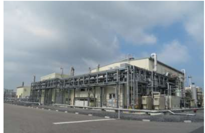
Appearance of building
