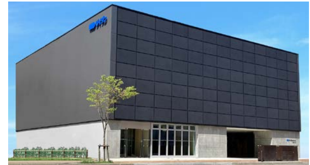
Enefice Hokkaido, completed in June 2021
