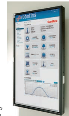
The monitor screen displays the current power generation.
