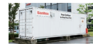
Power conditioner for the VPP demonstration installed in our Shiga Plant
