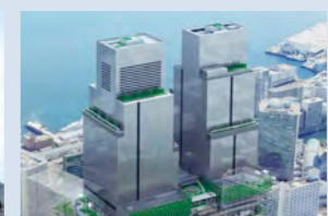
2021 Started construction of Shibaura 1-chome Project (South Tower)
