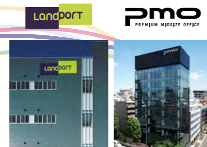
2007 Completed construction of Landport Atsugi
