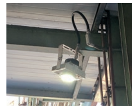
Newly installed lighting equipment
