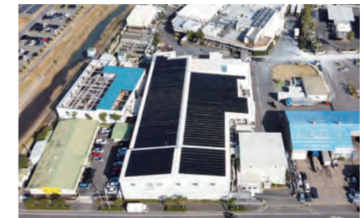
Solar panels at the Akune Plant of STARZEN MEAT PROCESSOR Co., Ltd.
