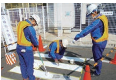
Painting zebra crossing on plant premises
