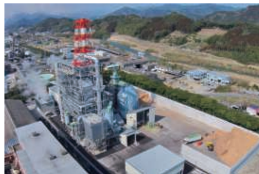
Biomass power plant (Oji Green Energy Nichinan/Miyazaki Prefecture)
