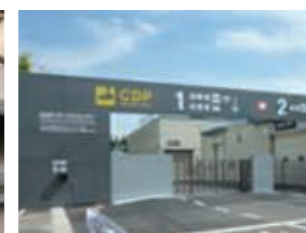
Confidential document processing facility (Oji Materia Edogawa Mill)
