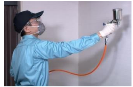
DUSKIN staff applying photocatalyst
