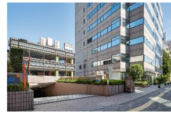
Indoor Drive-in Parking Lot
