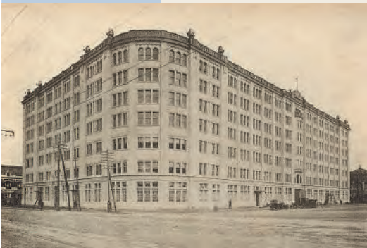
Tokio Marine and Fire Insurance Building
