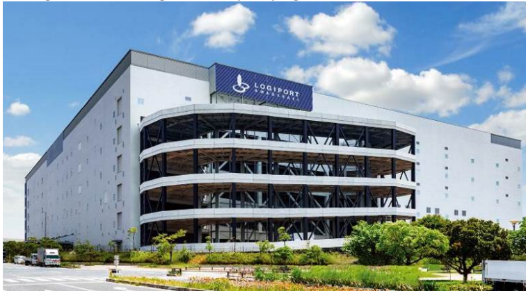
LOGIPORT Amagasaki (20 Ogimachi, Amagasaki-city, Hyogo)
