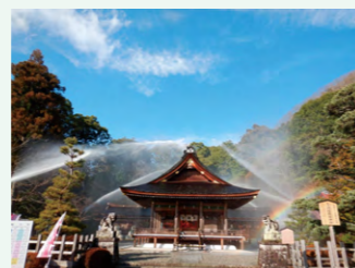
Fire extinguishing system for a cultural property (Nohmi Bosai)
