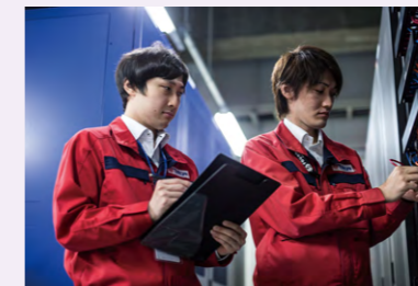
At Tokyo data center
