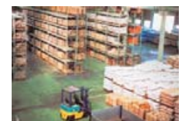
Kanto Logistics Center (Ibaraki Prefecture)
