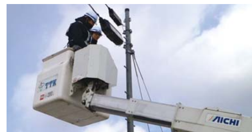
Students standing in the boom bucket of a bucket truck
