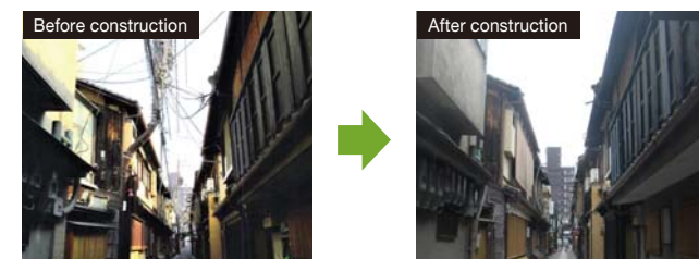
Construction to eliminate utility poles in Ponto-cho
