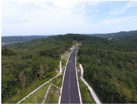
Route 45 Ube Ashigasawa area pavement construction work
