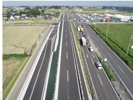
New Line 4 Koushu area pavement construction work (2020)
