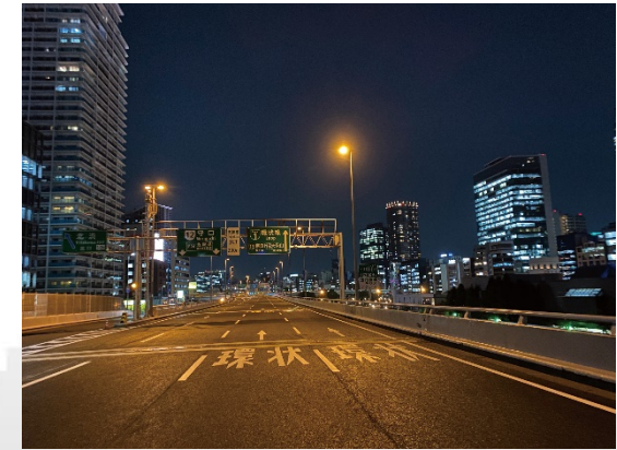
Large-scale pavement repair work (loop line road, January 2019)
