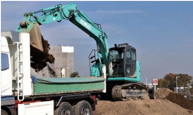
Automated operation trial for a power shovel.
