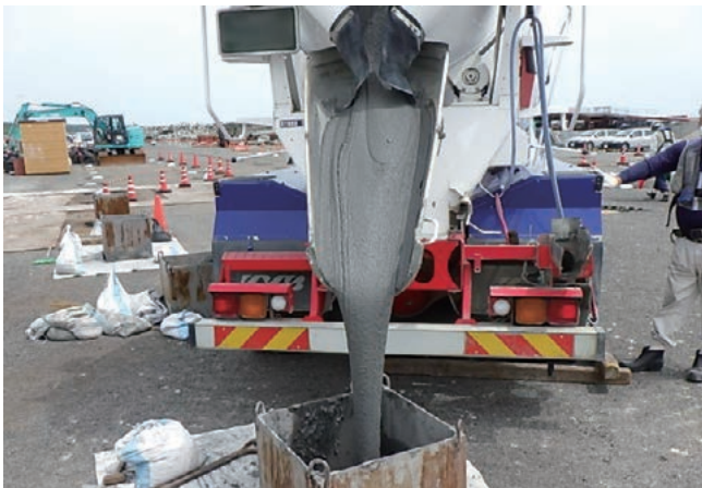
"Ash-crete" used to fill the interior of the mega float.
