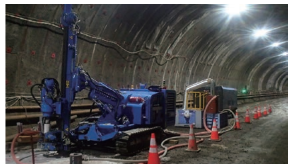
Trial construction in a tunnel.
