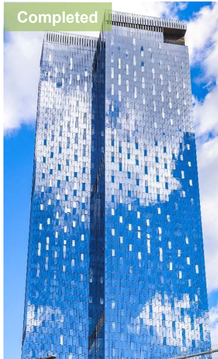
250 South Street (New York, USA) Total of 12 elevators
