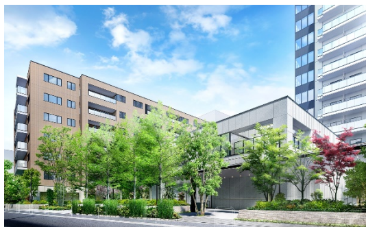
The Parkhouse Mita Garden Residence & Tower
