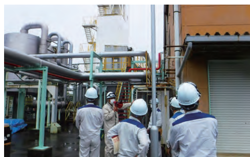
Executives conduct a safety inspection at the Yokkaichi Plant
