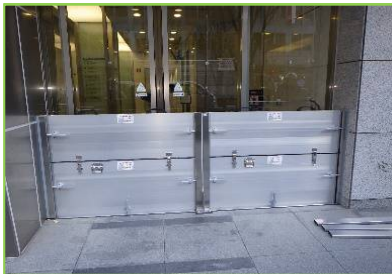
[Installation of tide prevention equipment] (NBF Higashi-Ginza Square)
