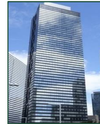
Shinjuku Mitsui Bldg. (Shinjuku-ku, Tokyo)
