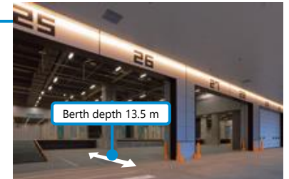
Truck berths are large enough to fit a whole 40ft container truck.
