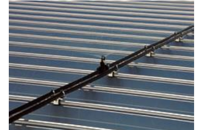
Facility has roof spraying system that uses well water to reduce the internal temperature.
